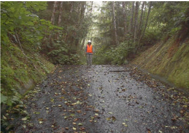
Top of concrete channel - summer flow
