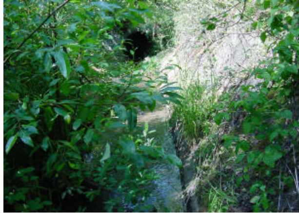
Highway Culvert Outlet (HUM299)
