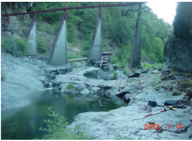
Upstream Debris Rack
