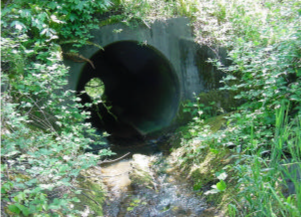
County Culvert Inlet
