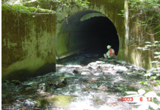
Culvert Inlet and debris blocker
