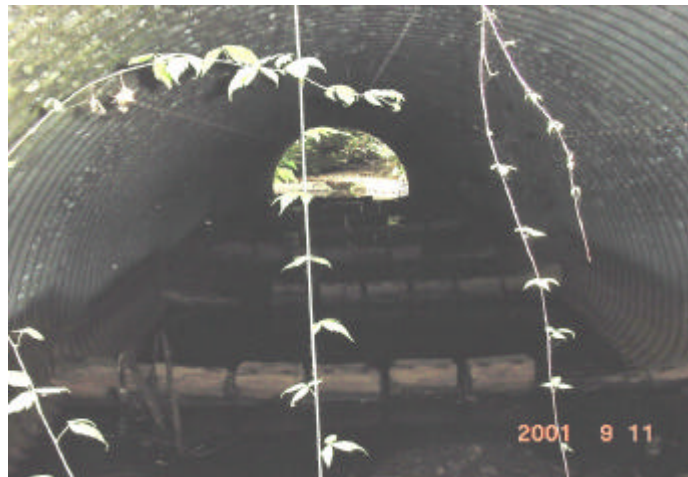
Wooden baffles in culvert
