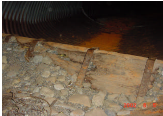
Weirs in Culvert 1
