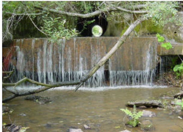
County culvert outlet (Essex Road)
