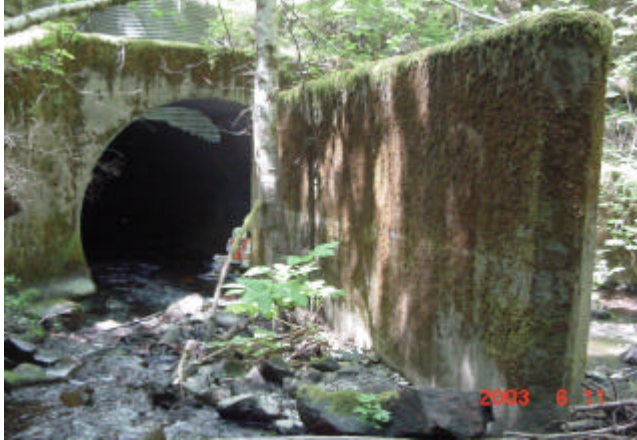
Culvert Inlet and debris blocker
