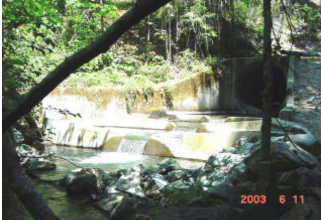
Culvert outlet and weir system
