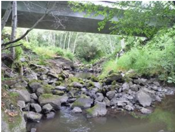
Figure 3. RSP partial barrier downstream of bridge – (Pre-treatment condition, 7/23/2013)
