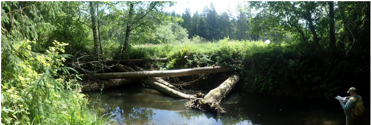
Figure 2. Trenched logs helped increase cover, provide high flow refugia, and bank stabilization (Post-Treatment Condition, 6/11/2019)
