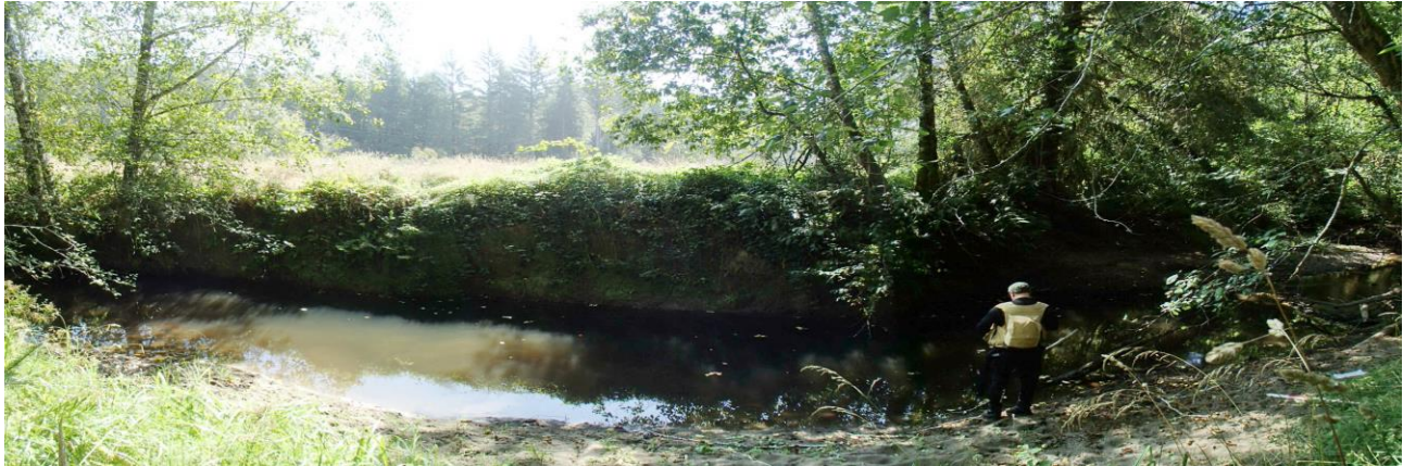
Figure 1. Unprotected, erosive bank at proposed site for LW structure placement (Pre-Treatment Condition, 8/18/2016)
