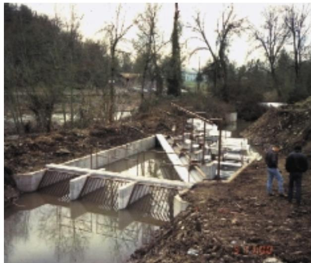
The four-bay screen in Figure 4 is for flows up to 25 CFS and costs \$45,000 to construct. This was a joint project, with an ODFW crew doing most of the concrete and metal work. Trout Unlimited paid for some of the costs, and some labor and equipment (dump trucks) were donated.
