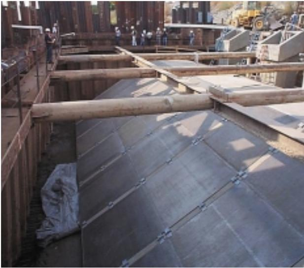
**Figure 9. Airburst screen cleaning system**
