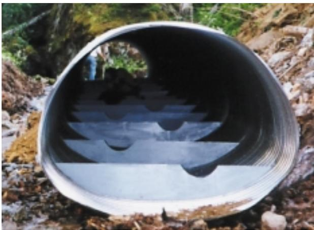
**Backing Water into the Culvert (Drop Structure)**
