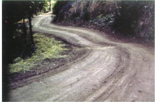
culvert might fail. The water then would go into the rolling dip and across the road where we direct it off on an armored down spout, or an energy dissipater at the indigenous soil/nick point of the fill. With that armored, if a failure occurs, we're less likely to lose the entire fill.
