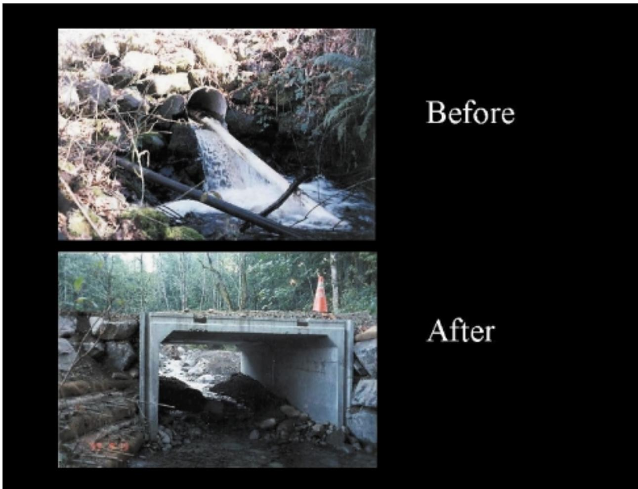
**Figure 9. Looking downstream from the new culvert at the rebuilt reach of O'Grady Creek after construction. The streambed here is about three feet higher than the eroded streambed. Buried boulder wedges create a stepped reach of pools for fish passage. LWD was added for habitat diversity.**
