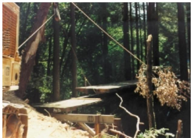
cannot carry nearly the load of a railroad flatcar with its big deep I-beam, although boxcars are good for really short spans.
