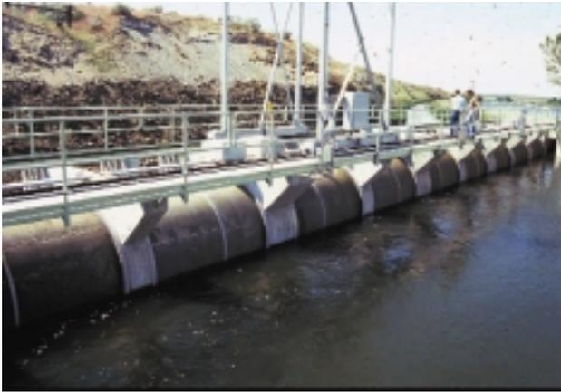
motors turning the drums. Water flows along the screen faces into the bypass. Electric-powered drum screens can be very large, as shown in Figure 6.
