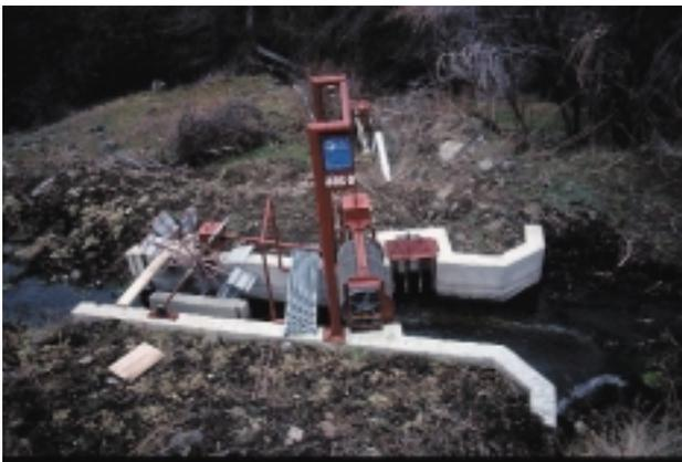
Generally we install small screens as in Figure 3, which cost \$4,000–\$5,000 per CFS. The screens are powered by paddle wheels because there is often no available electricity. Water enters the structure, turns the paddle wheel, gets reversed through a couple of gearboxes, and then goes to the drum. The drums all turn in the same direction and are very well sealed. The fish enter a bypass that carries them safely back to the stream.
