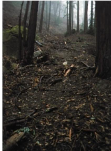
Tractor-crushed debris works perfectly (Figure 5), eliminating the need for straw bales or other imported material. One excavated crossing was an old log crossing. We incorporated the wood back into the design of the removal, leaving large woody debris (LWD) in the area of influence, although not within the stream zone itself (Figure 6).
