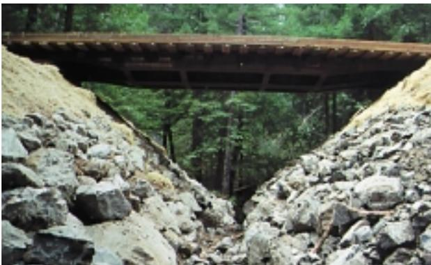
be suspended. The bulldozer pulls across the cavern to be spanned instead of pulling down to the creek and up the other side and tearing everything up. We suspend these with the bulldozer and then set them in place on either side. However, this process is complicated if the site is on a bend.
